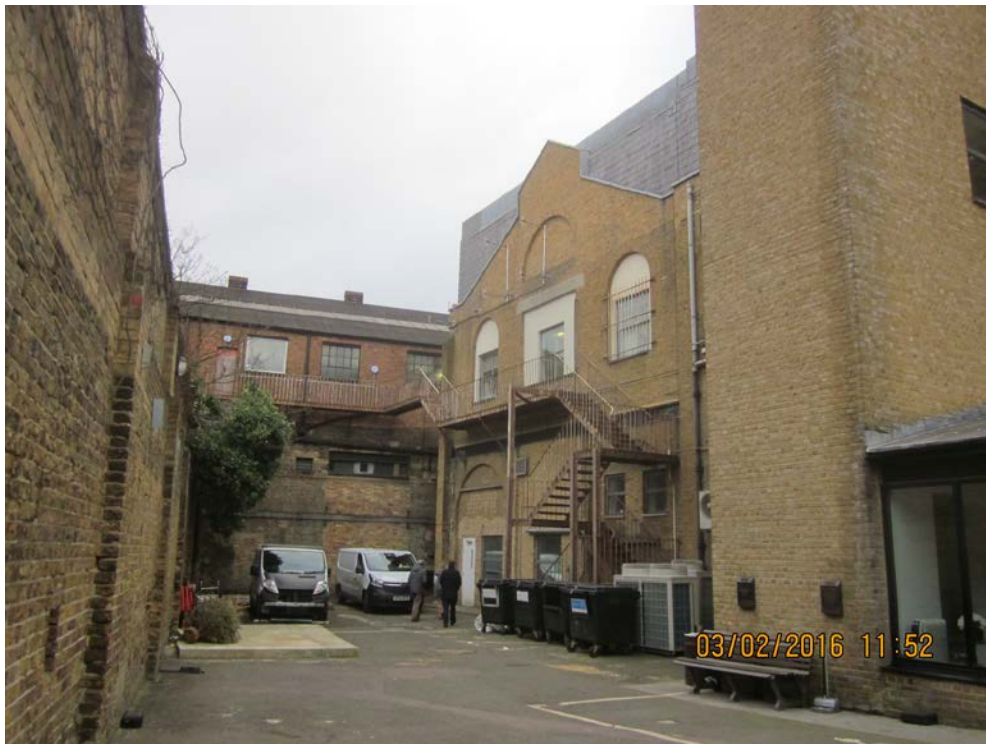
Rear of 25 Eccleston Place
